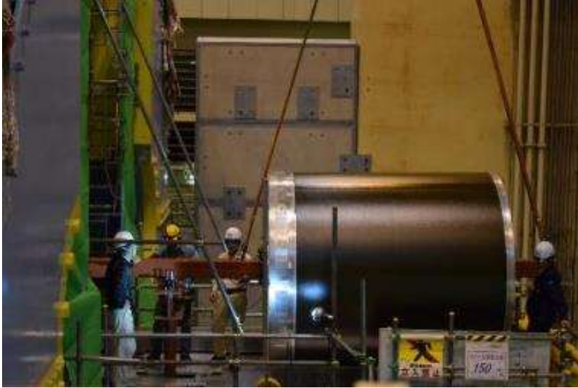
Installation into Belle II structure with inner bar without touching Barrel PID
