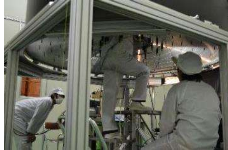
One person could access inside to string wires.
