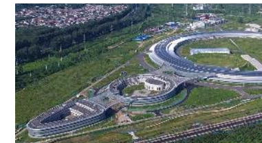
Nov. 3, 2023 Civil Construction for ancillary buildings completed
