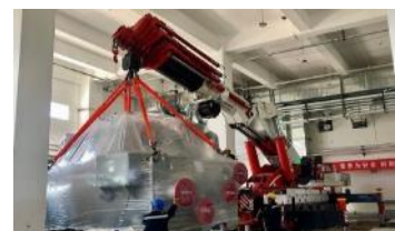
Apr. 13, 2021 Utility installation in NO.2 Hall commenced
