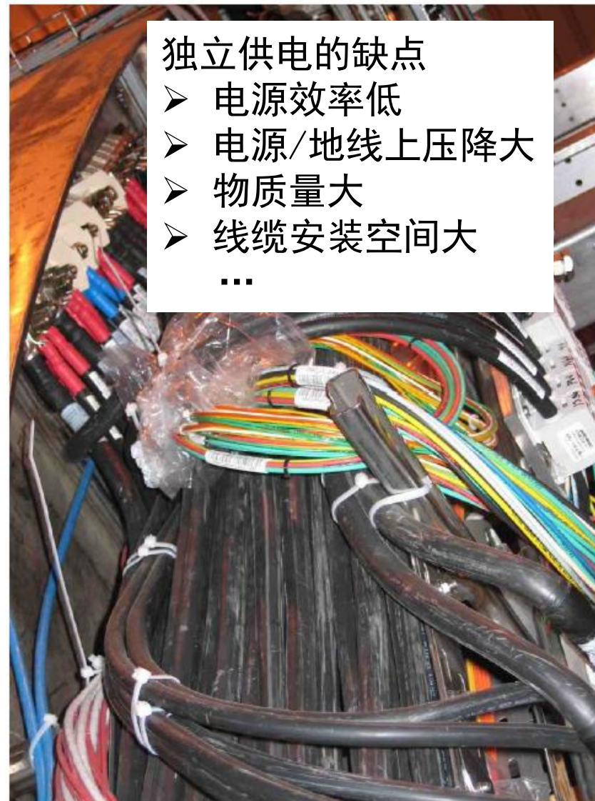
Figure 9.19: Cable tray showing low voltage cables and distribution boxes on CalFrame.
