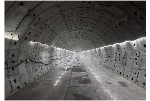
Eastern tunnel between Shaft #4 and Shaft #5
