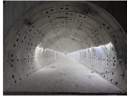
Eastern tunnel between Shaft #3 and Shaft #4
