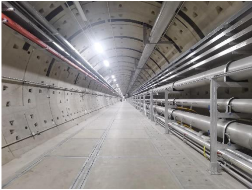
Tunnel between Shaft#1and Shaft #2
