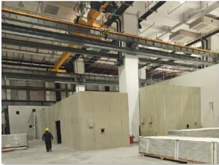
Constant temperature shed completed
