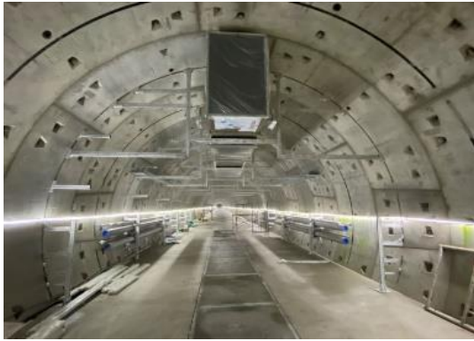
Eastern tunnel between Shaft #2 and Shaft #3
