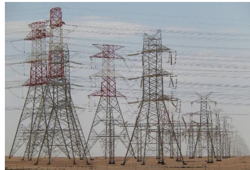
Electric power transmission
