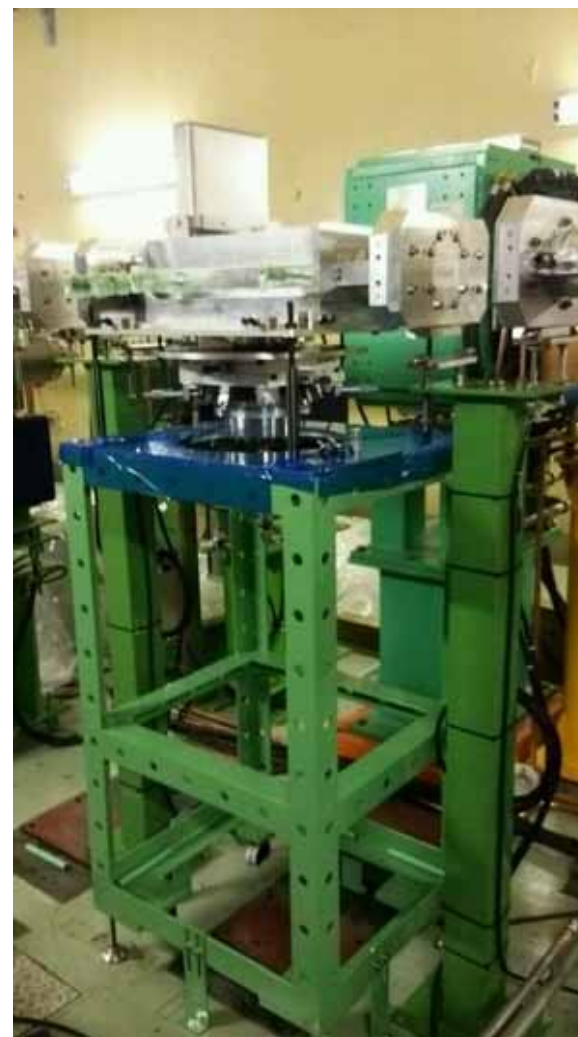
Extraction chamber installed in tunnel. (Vac. Group)
