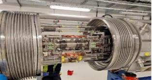
First interconnection of a pair of dipole modules in the accelerator tunnel, executed by IFJ PAN Krakow
