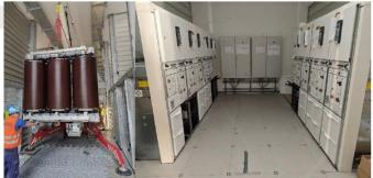
Installation of transformers and switchgears of the main power supply of the Dipole-Quadrupole Magnets completed by GE Vernova. Germanv
