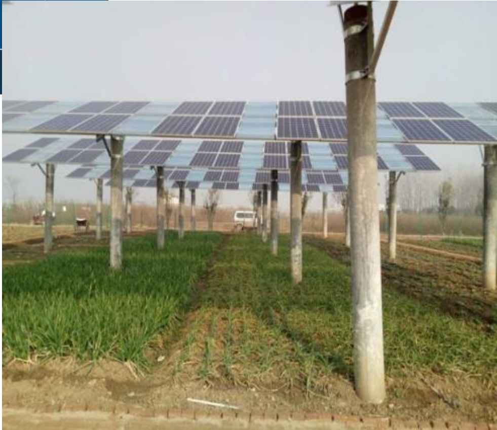
With the novel design methodology, the panels are placed at a height of at least 2.5 m from the ground. Image: University of Science and Technology of China
